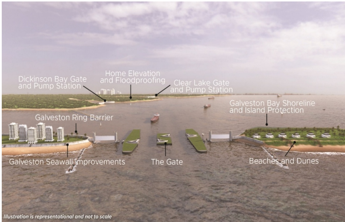
Figure 7: Conceptual rendering of the Galveston Bay Barrier System.
